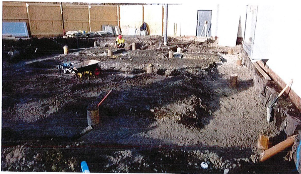
Reduced level dig to extension classroom and blinding to new ground beams. Pile heads visible.
