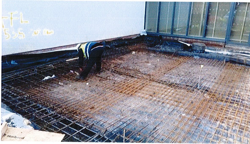
Infill classroom area with steel reinforcement structure to floor and DPM to perimeter.
