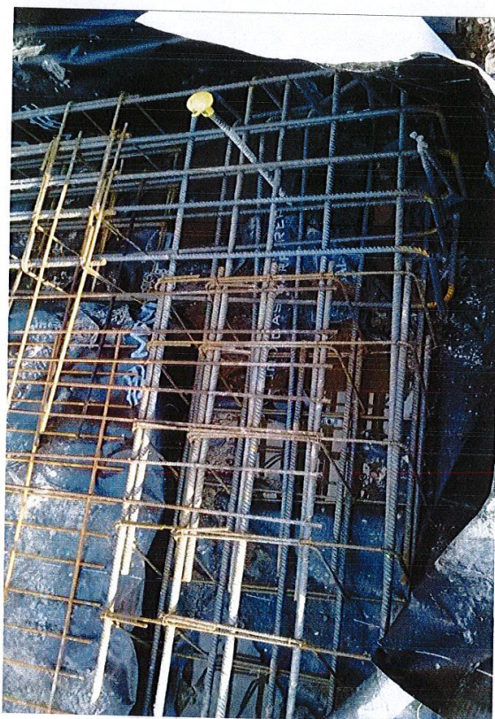
Steel reinforcement to foundations
