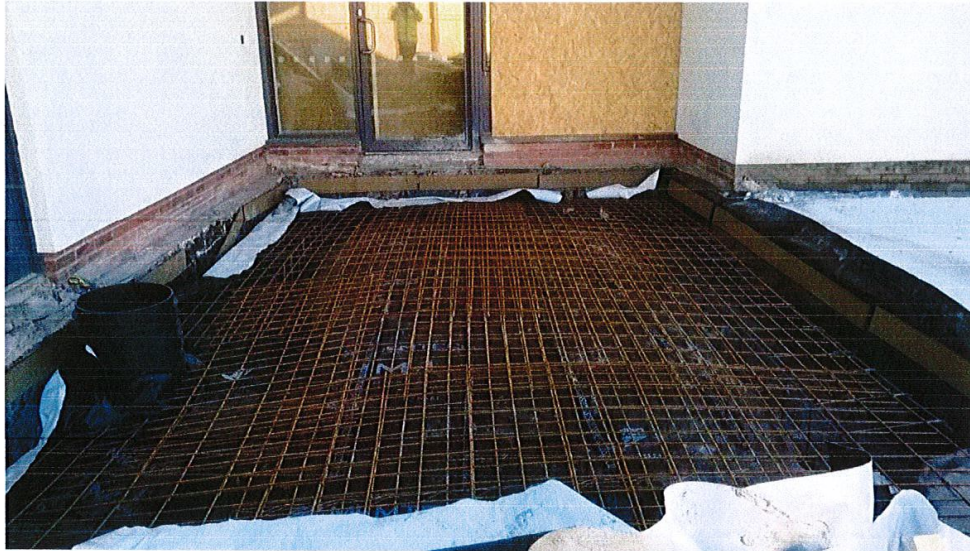
Floor slab steel reinforcement outside the redundant rear entrance.
