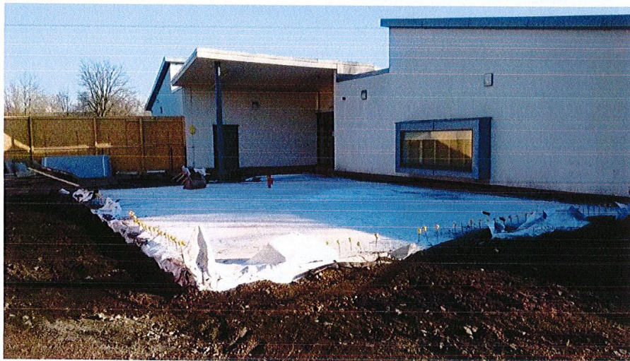
Concrete slab to extension classroom including foundations and floor.
