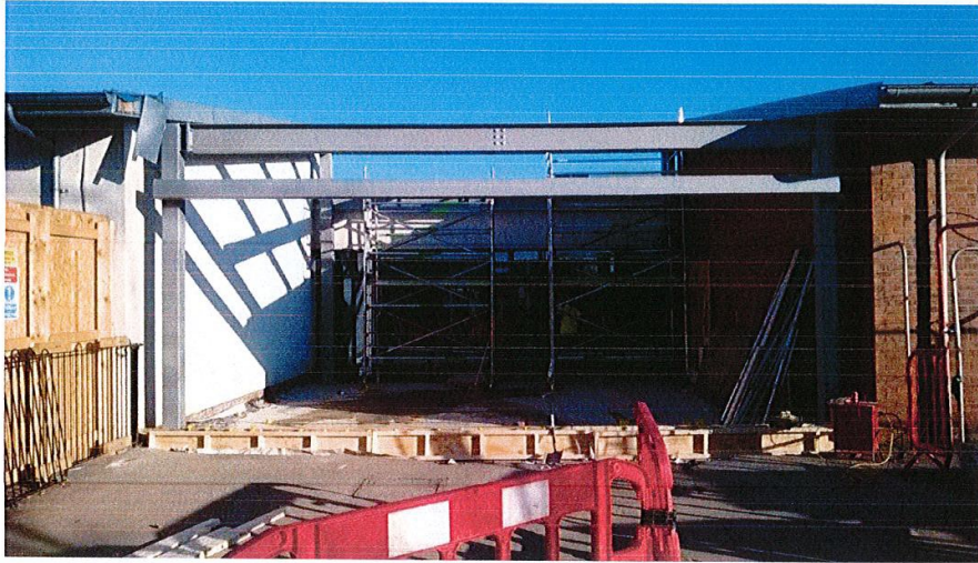
Infill classroom area with concrete cast to foundations and slab together with superstructure.
